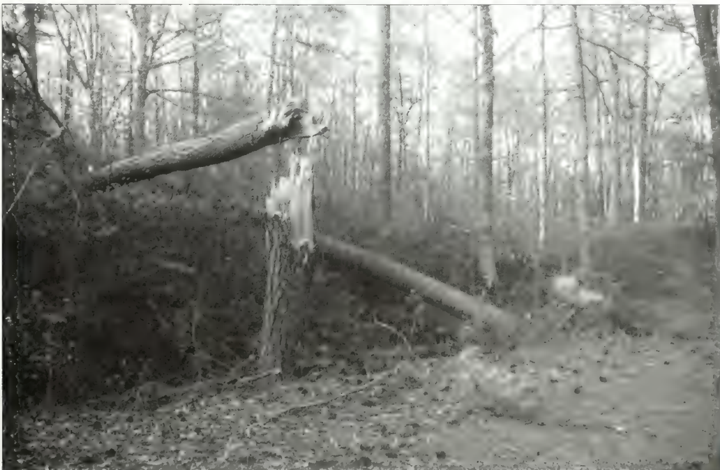
Figure 5.6. Storm-thrown tree, Union Fort Fisher, Petersburg National Battlefield. Permitting large trees to grow on engineered slopes, increases risks that wind, could topple the tree and displace a large volumes of the earthwork with its roots. Falling trees also pose impact risks to structural features (Olmsted Center, 1998).
